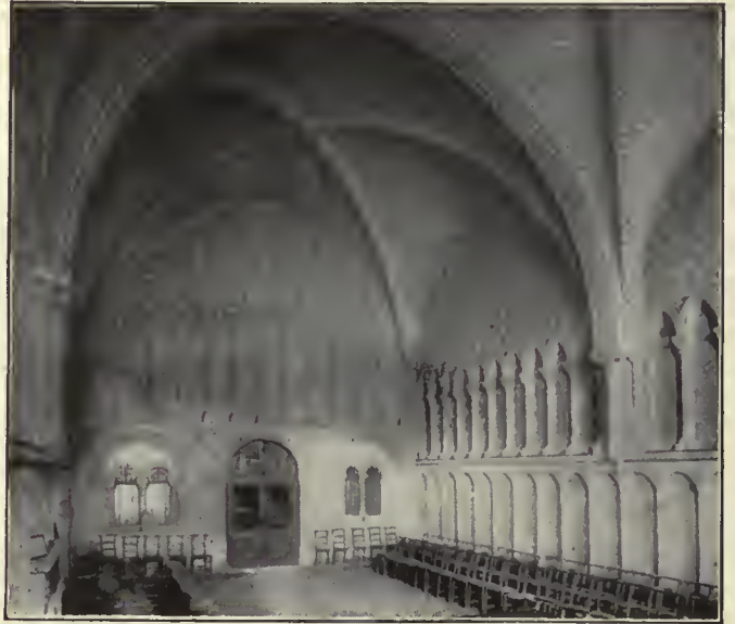
Photo, Valentine & Sons. FIG. 14.—INTERSECTING RIBBED VAULTING. Late example. Chapter House, Bristol Cathedral.
